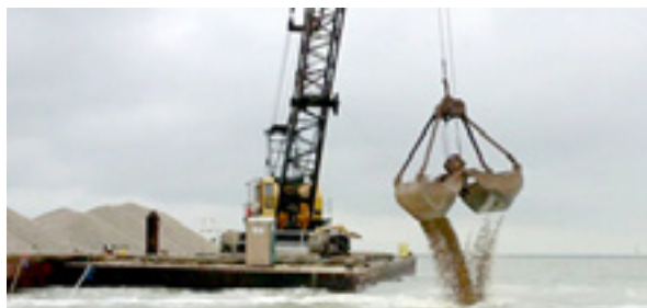
The deployment of oyster shell substrate on the constructed oyster beds
